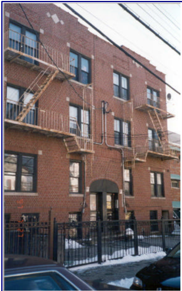
3940 Barnes Avenue in the Williamsburg section of the Bronx has 32 apartments and $896,978 of mortgage insurance from REMIC.
