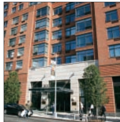
Court House 321 Apartments Downtown, Brooklyn
